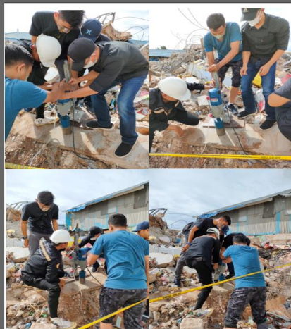
Proses Coredrill Kolom Beton
